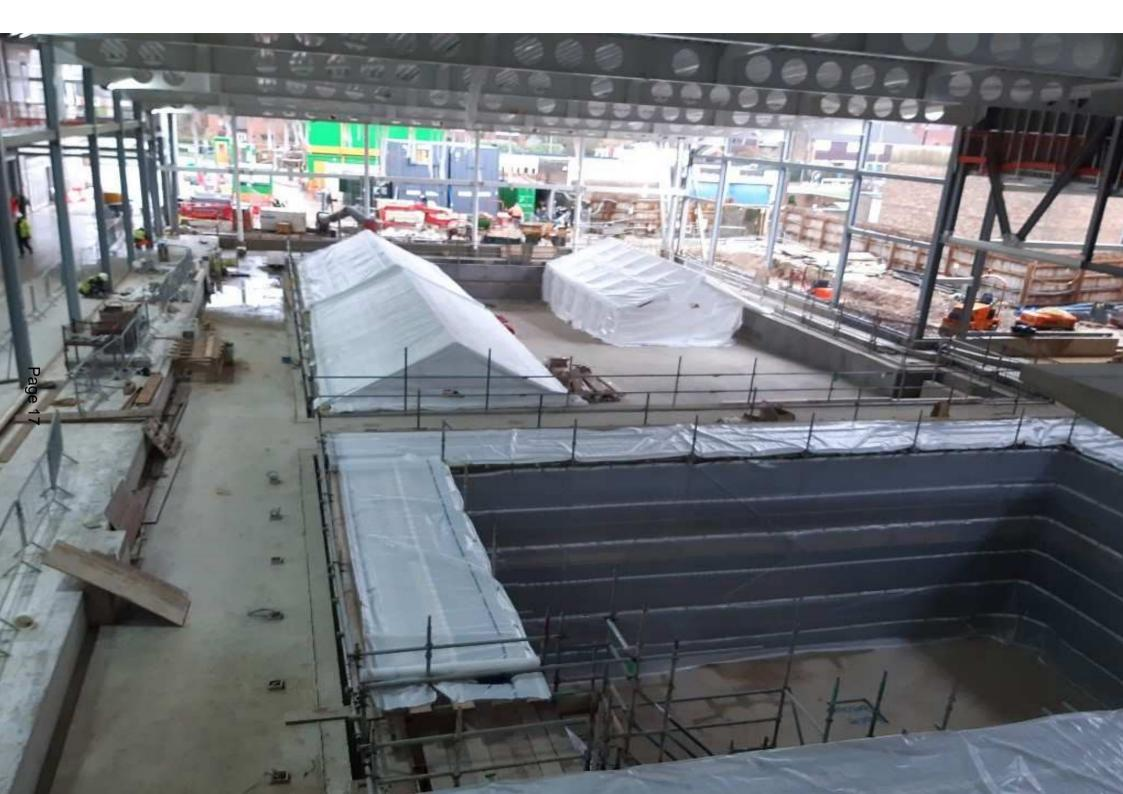
The building sub-structure including the swimming and diving pools has now been completed. This also includes all underground drainage.
